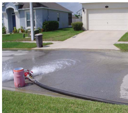
Unidirectional flushing at a Melbourne neighborhood.
