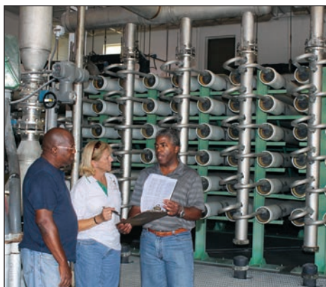
WATER PRODUCTION staff members were selected as Melbourne's water was selected as best in a regional competition. Pictured is the filter array that is involved in processing of well water.
