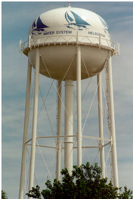
Elevated water storage tank in Indialantic.
