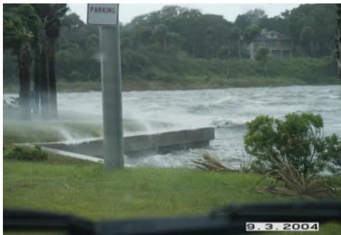
The first of last year's storms to wallop Melbourne was Hurricane Frances, shown here beginning to stir up the lagoon at the Melbourne Causeway.
