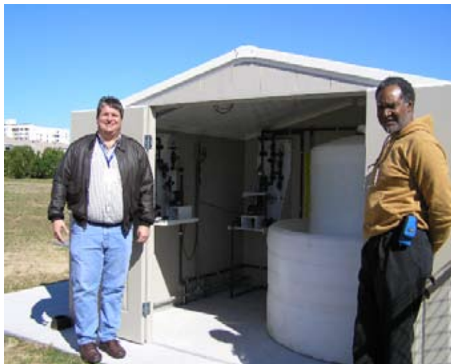
Assistant Water Production Superintendent Dave Phares (l) and Electronics Technician Vaughn Curry stand in front of new structure installed at the Canova Beach Pump Station.
