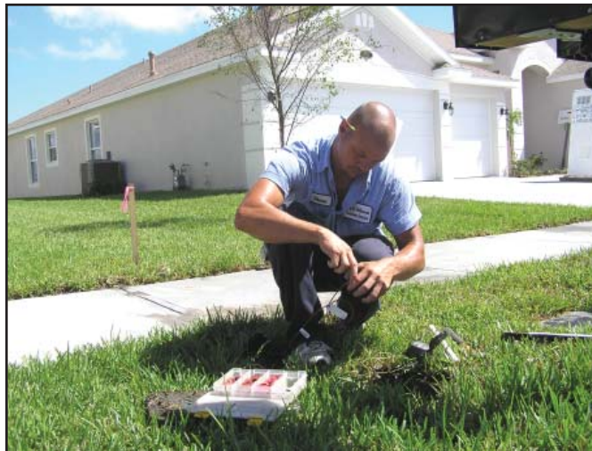
Shane Robbins installs automation equipment to convert meter.
