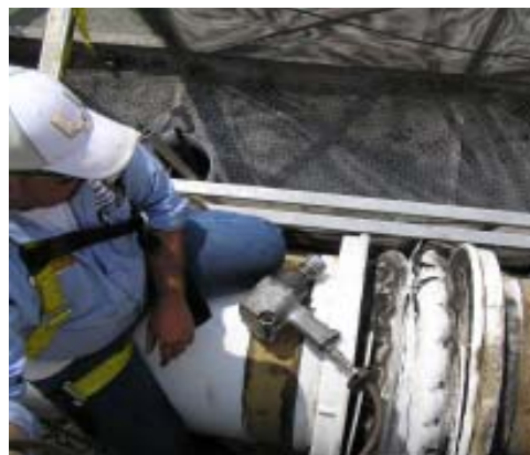
Robert Sigman works on repairing the damaged expansion joint.
