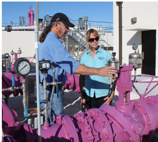
Blankman (left) and McDonald discuss improvements at the Grant Street WRF.
