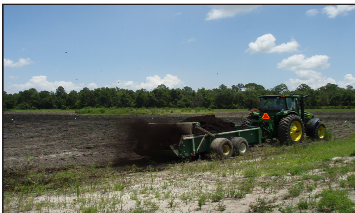
Melbourne's ferric residual is being applied with a manure spreader over the top level of soil at the future wetland site in Palatka.
