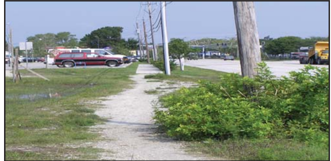
Section of sidewalk, partly paved and partly dirt, on the south side of Aurora Road.
