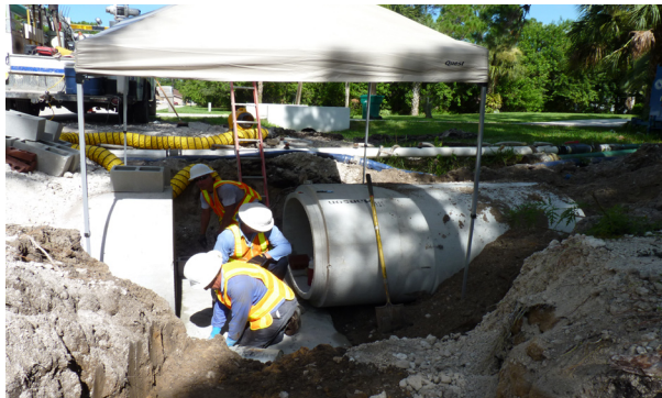
Working on the project, from back, are Shane Buckelew, Josh Baker, and Luis Burdett. Not pictured are Joel Mendolia, William McDonald and Foreman Joe Gervais.
